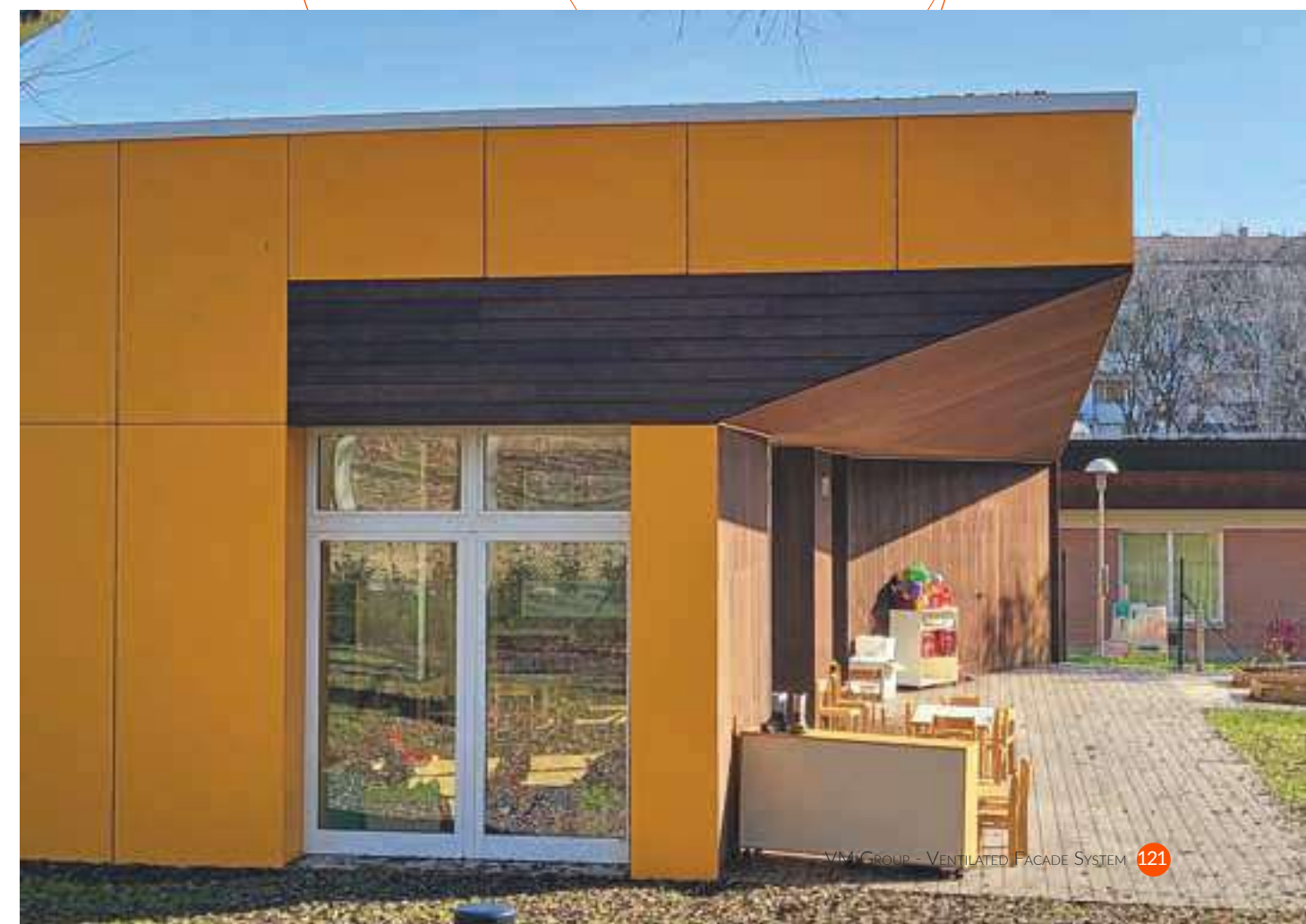
BOLOGNA Construction of the ventilated facade of a nursery school in HPL with concealed fastening.
