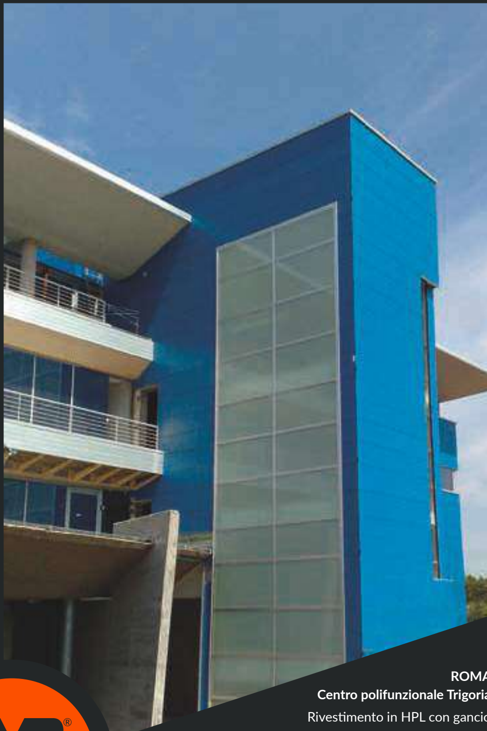
ROMA Multipurpose Trigoria center HPL cladding with hidden hook
